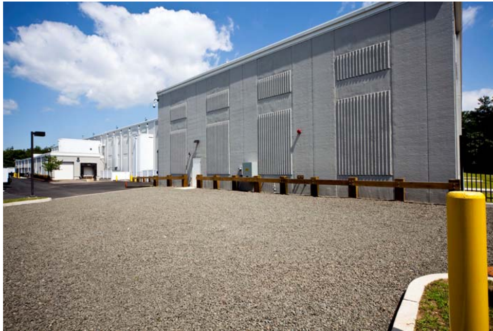
Yale University Storage Facility (view from the north) Source: Photo provided by Michael DiMassa, Director of YUSF
