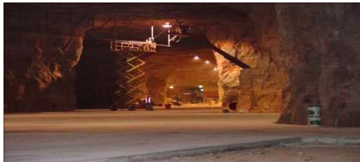
NARA facility (constructing storage bays) Source: NARA
