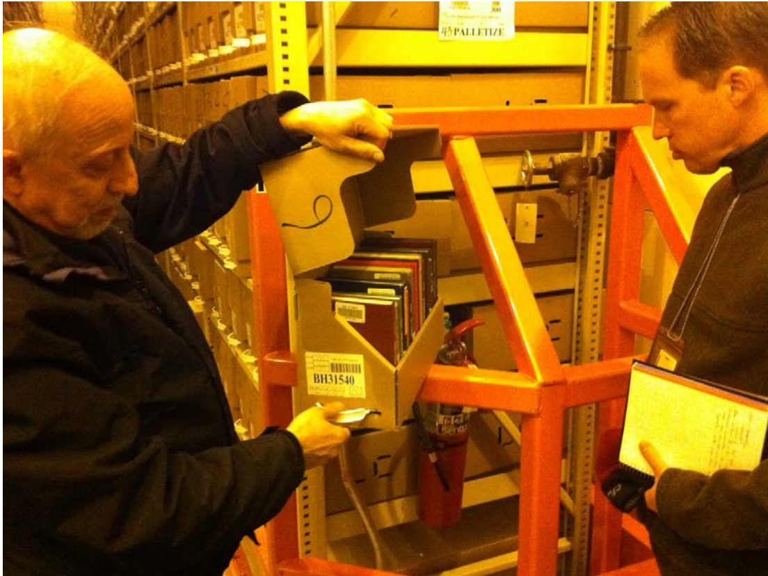
Library of Congress High Density Storage Facility (covered box) Source: Photo by Seth Elan
